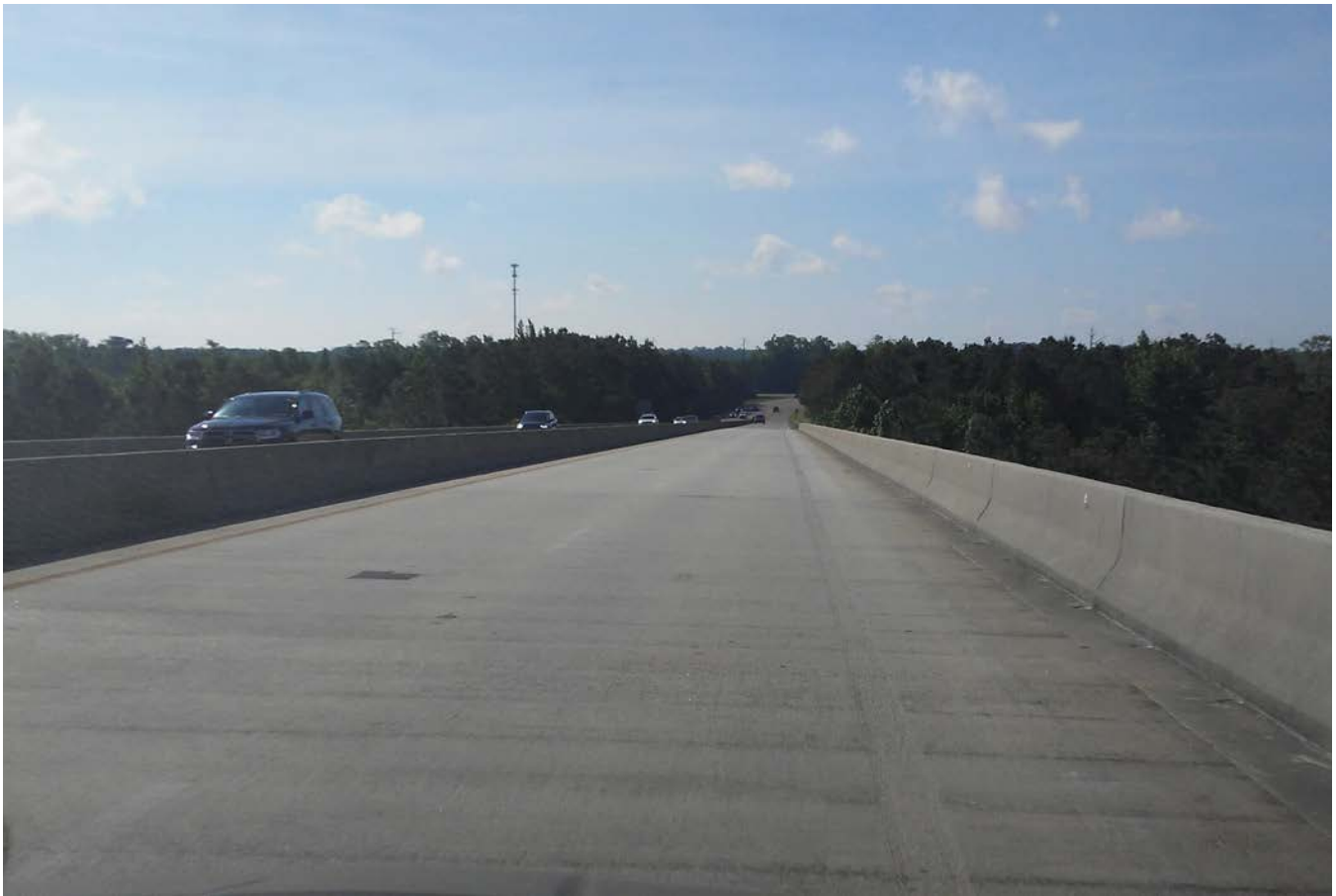
A view from the top of Joseph P. Knapp Bridge reveals limited space to provide pedestrian facilities across the Intracoastal Waterway.
